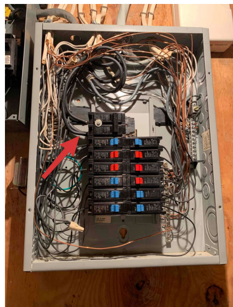
Circuit breaker manufacture prohibits double tapping of this model
