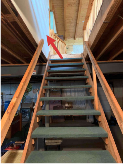
Improper handrail
