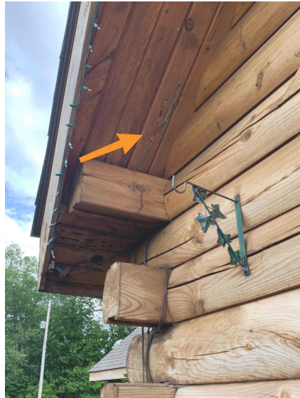
Carpenter bee type damage
