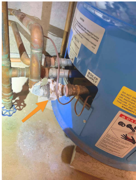
Corroded connections are prone to failure
