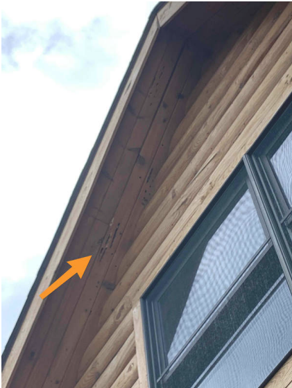
Carpenter bee type damage
