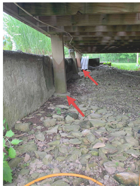
Front deck support posts show signs of movement
