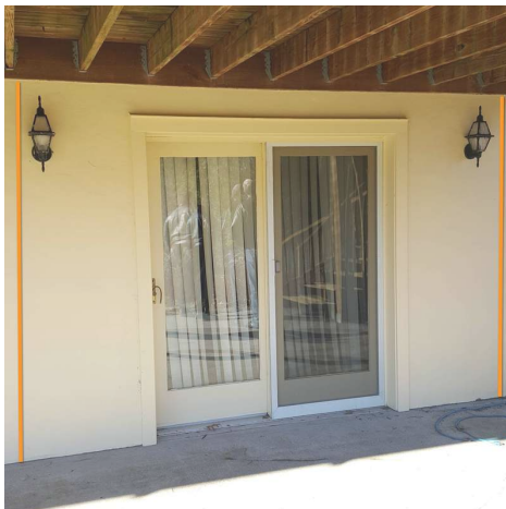
Wood framing and stucco extends beyond the light fixtures.
