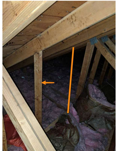
Arrow indicates added support. The line indicates missing support
