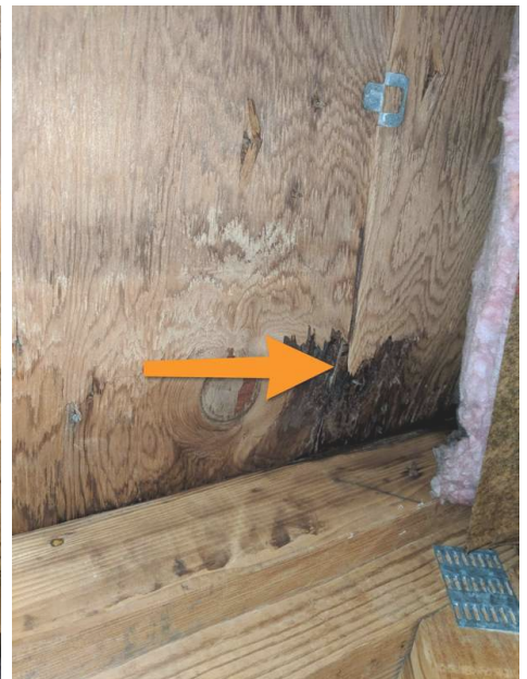
Cracked Sheathing
