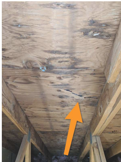
Cracked Sheathing
