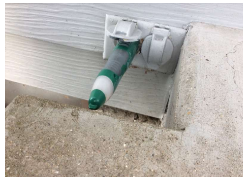
Not GFCI ProtectedWest Exterior
