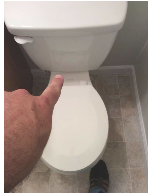
Toilet Loose Downstairs Half Bathroom
