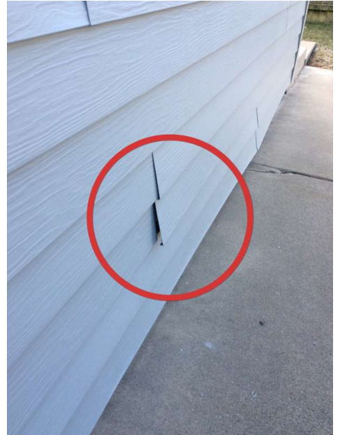
Loose Vinyl SidingWest Exterior
