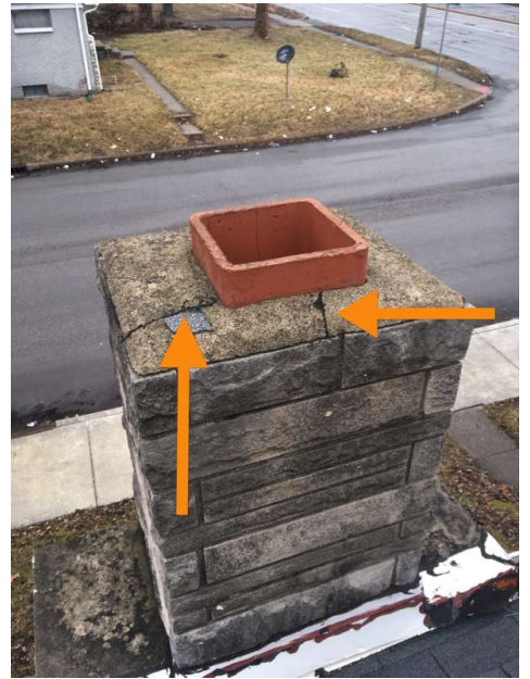
Cracked Chimney Cap
