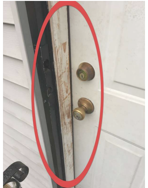
Deteriorating/Missing PaintGarage Exterior Door
