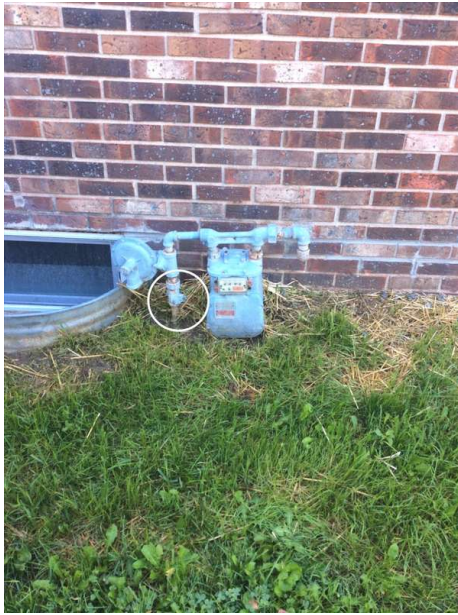
Main Gas Shutoff
