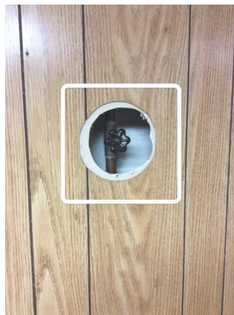
Main Water Shutoff
