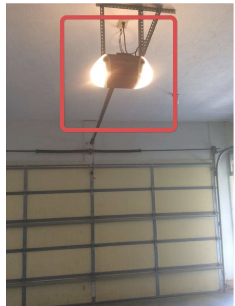
Safety Reverse Needs Adjustment Garage Exterior Door
