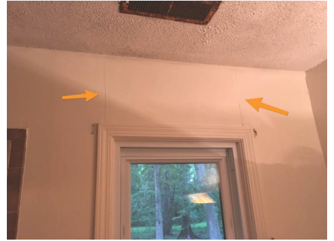
Example, multiple areas throughout the home exhibited these cracks
