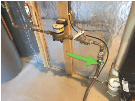
Main Shut Off Valve
