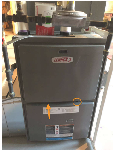
Left one missing, Right One OK
