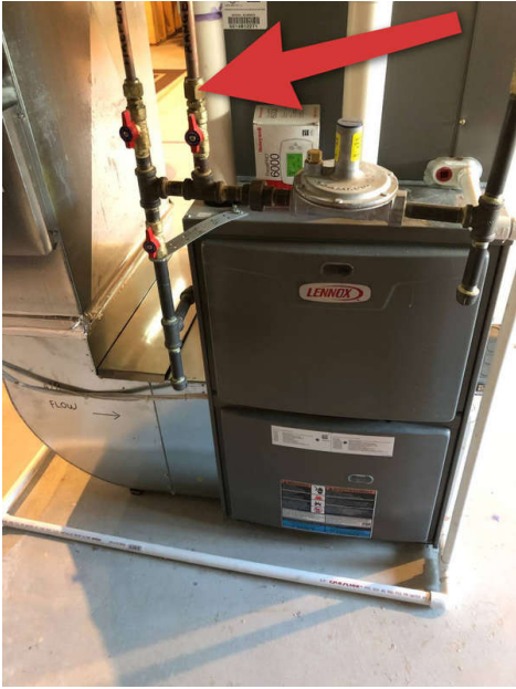
Gas leak area
