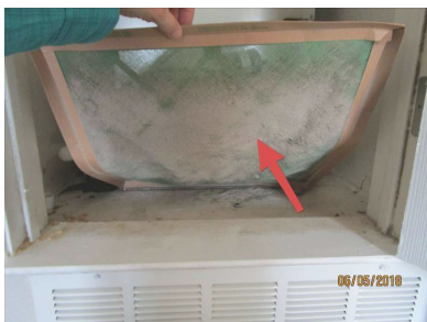
A/C filter dirty and flimsy.
