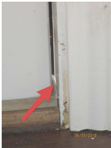
Noticeable gap on bottom (right) of back door.
