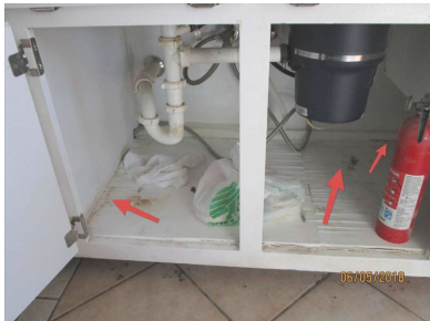
Wood cabinetry under the kitchen sink shows signs of previous water damage.
