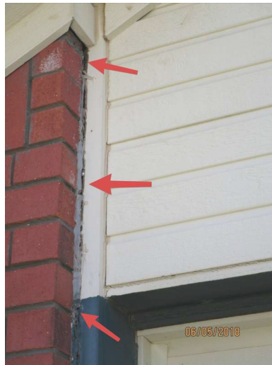
Caulking around multiple windows is dry rotted. This photo taken in front (East side) of home.
