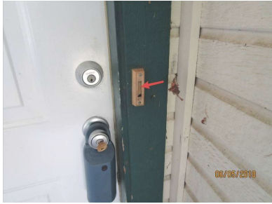
Doorbell does not function properly.
