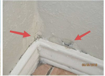
Drywall shows signs of previous water damage (master bedroom closet on wall opposite side of sinks)
