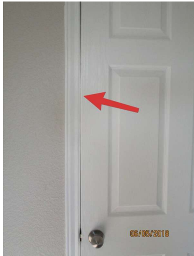
Door sticks when opening and closing. (This pic is in Northeast bedroom)
