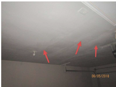
Drywall on ceiling in garage is sagging in multiple locations.
