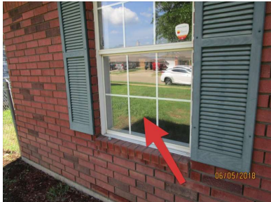
Window screen missing (Southeast corner of home facing street)
