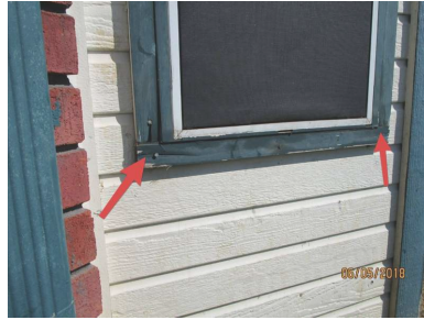
Trim around window shows signs of water damage. (Northwest corner of home)
