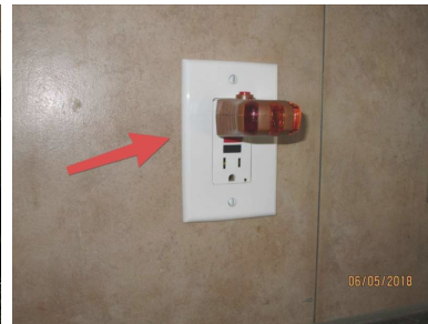
No electricity detected at GFCI receptacle to the "left" of kitchen sink.
