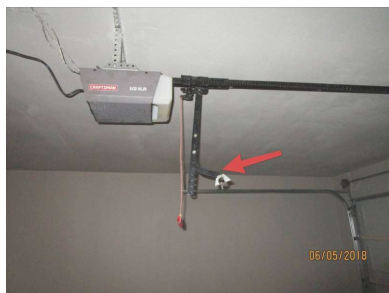
Garage door opener disconnected.
