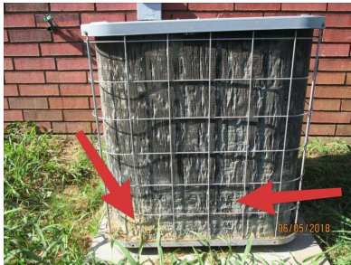
Condenser unit fins in very poor shape.
