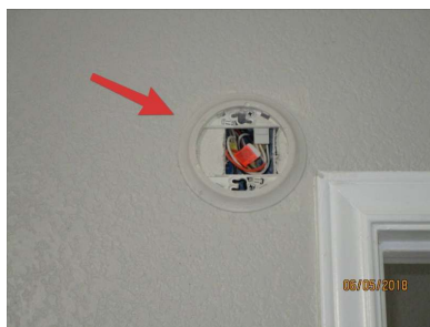
Smoke detector missing (front bedroom to "right" of front door).
