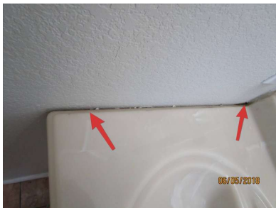
Gap between wall and sink in master bathroom.
