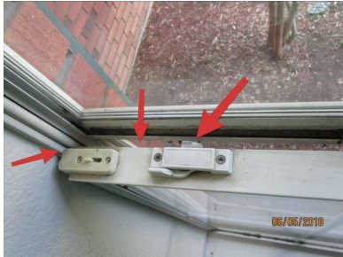
Window in front bedroom (right of front door) is out of adjustment, and cannot be secured.
