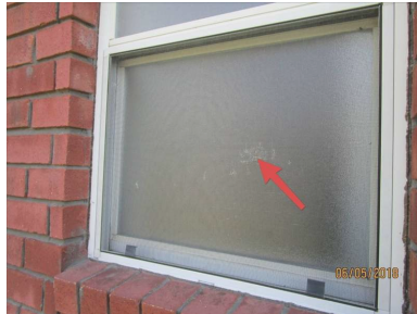
Multiple screens have holes in them (this is on North side of home)
