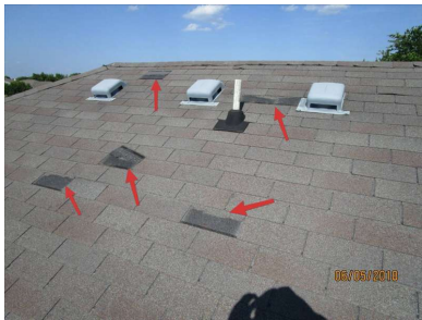
Numerous shingles missing, and other shingles not laying properly. (this pic is on West side of roof facing backyard).
