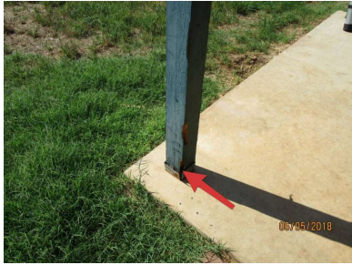
Support column on back patio shows evidence of water damage.
