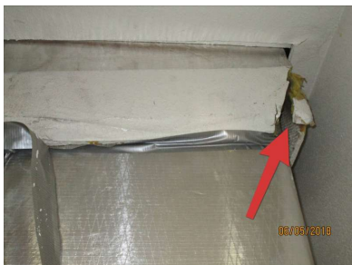
Duct system (above evaporator unit in HVAC closet) not sealed properly.
