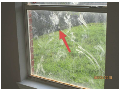
Glass is cracked in window (Southwest bedroom)
