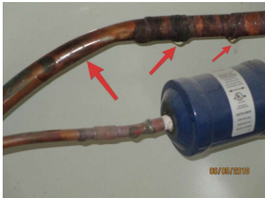
Insulation missing from Suction line, and line is "sweating." (this photo taken in HVAC closet on inside of home).
