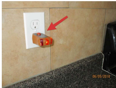
No GFCI protection detected (outlet left of stove).
