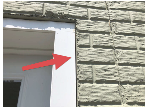
Rear Basement Door
