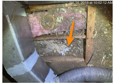
Missing attic insulation.
