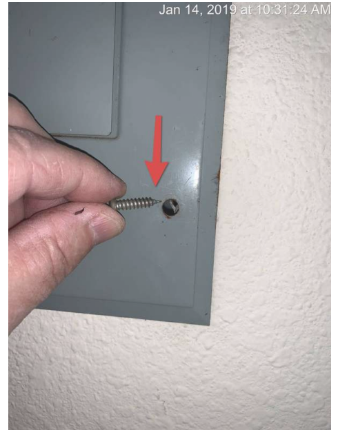
Sharp screws used to install panel cover.
