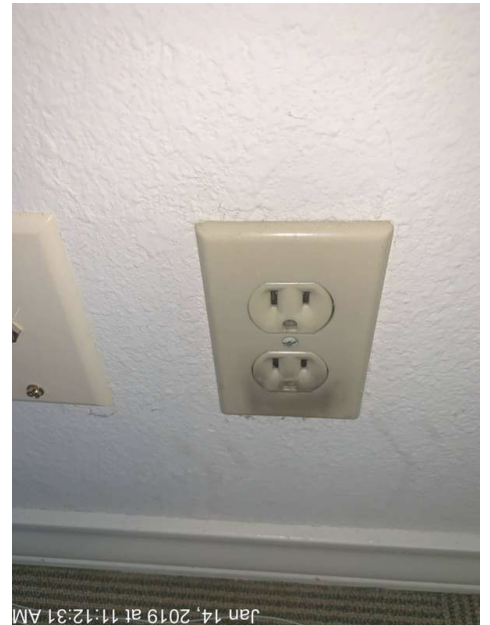
Overheated Receptacle.
