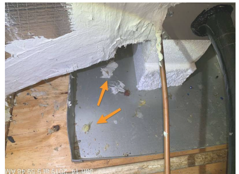
Debris in condensate pan should be cleaned.
