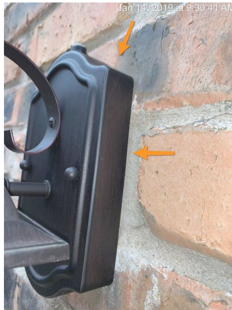
Seal to prevent water intrusion.
