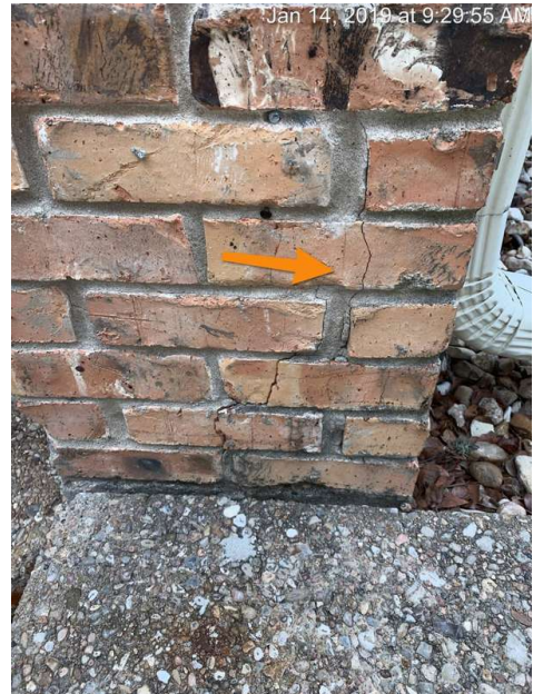
Minor cracking in brick veneer. Recommend monitoring to determine if any additional movement is occurring.
