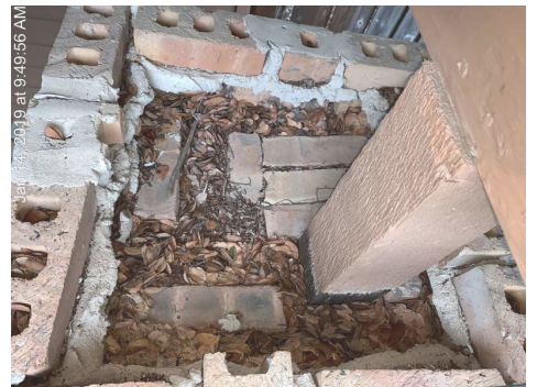
No cap for brick column.
