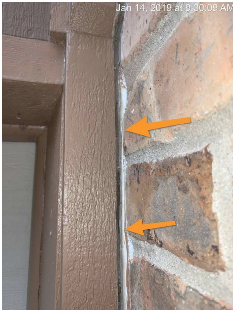
Seal to prevent water intrusion.
