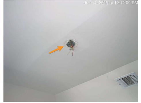
Fixture missing leaving exposed wiring.
