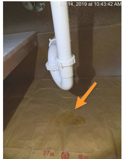
Bar sink leaking.
