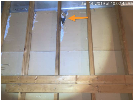
Opening in draft stop
