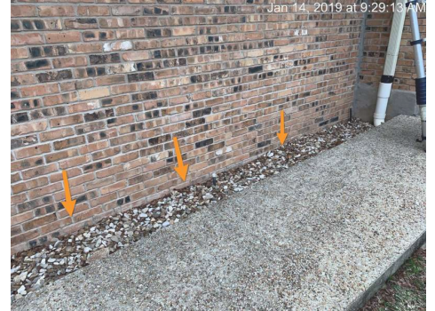
Should be 4-6' inches of foundation visible.
