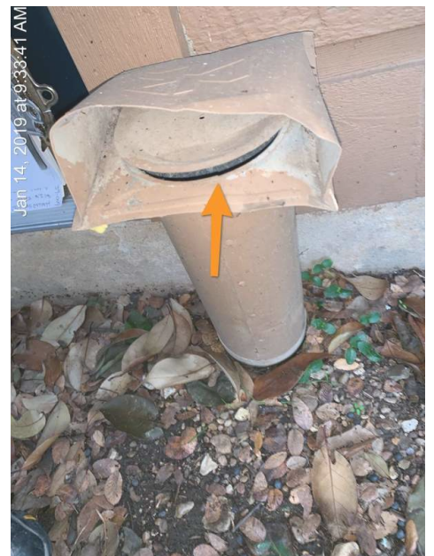
Flapper on dryer vent not closing. Recommend replacement.
