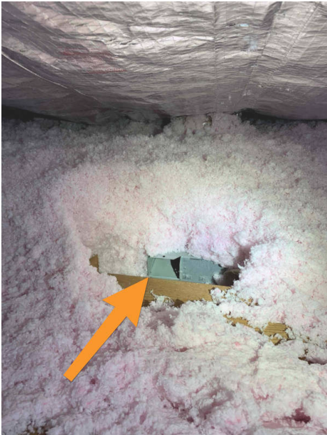
Guest Bathroom Front part of home
