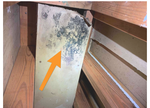
Access panel behind shower wall in MIL Bathroom
