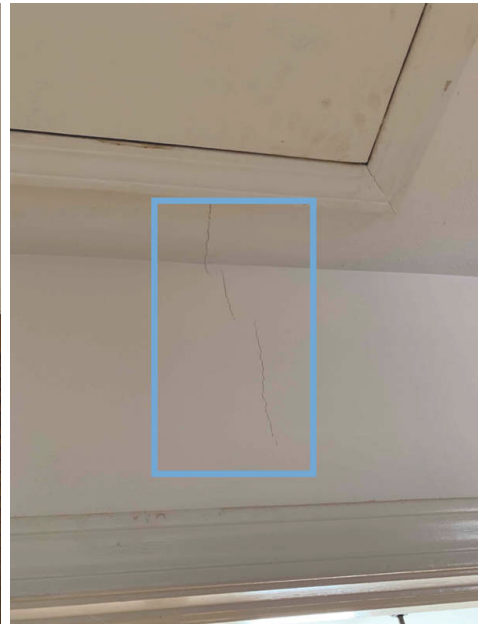
Front hallway by attic access
