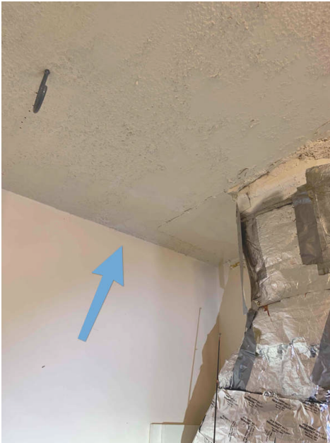
Back storage room
