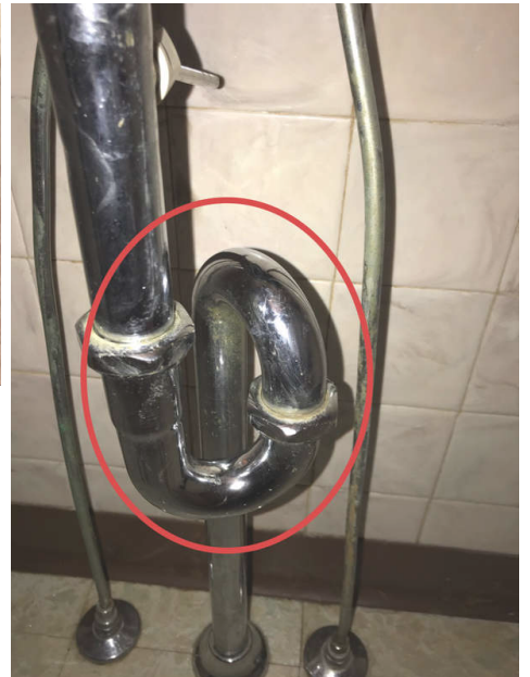
2nd Floor Bathroom
