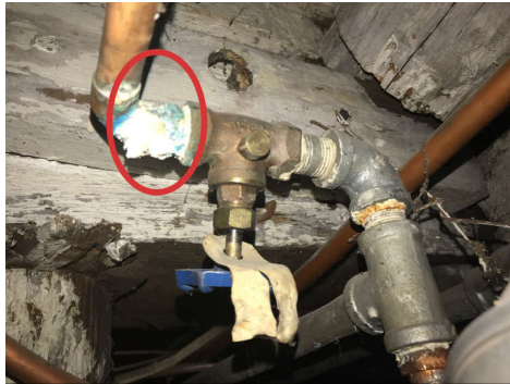
Above Water Heater
