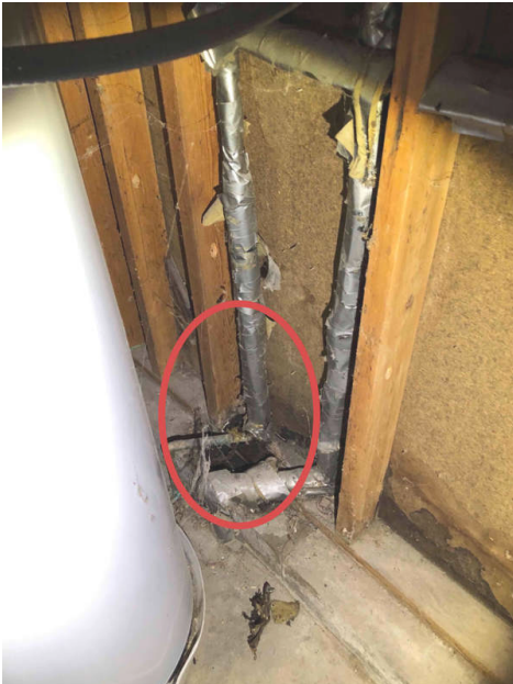
Hot water pipe Garage
