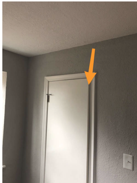
2nd floor Bedroom Left
