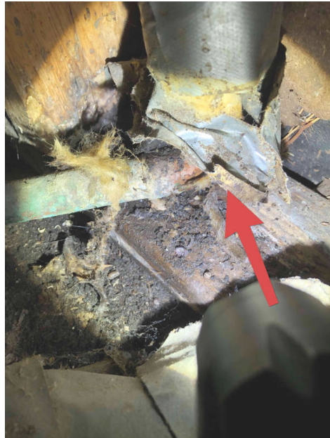
Wet/leaking hot water pipe Garage
