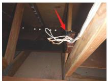
The electrical wires for the garage attic ceiling light switch are showing a sub standard installation.Excessive wires exist which are not sealed properly at the switch box.Repair is needed.
