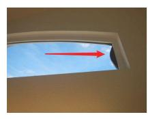
The right side picture window weather gasket is damaged.Repair/replacement is needed. Recommendation Contact a qualified professional.
