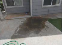
Standing water observed, which could indicate poor drainage and/or grading. Recommend monitor and have looked at by a concrete specialist.
