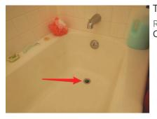
The tub's drain stop is missing. We recommend it be replaced.
