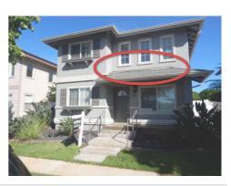
Flashing is loose. Needs nailed down and caulked. Recommend further evaluation from a licensed Roofer.
