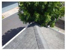
Tree debris observed on roof. This can cause improper drainage to gutters and downspouts. Recommend clearing debris.
