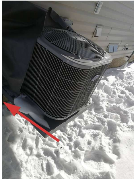
Ac unit attached to the foundation.
