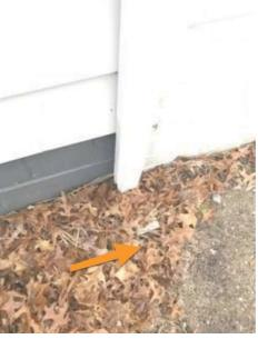
2.2.3 Roof Drainage Systems **DOWNSPOUTS MISSING**
