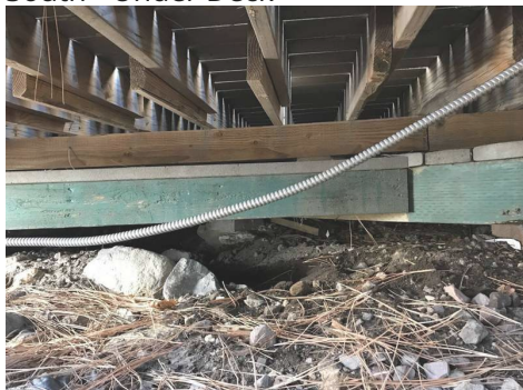
South - Under Deck
