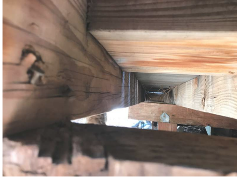
South - Under Deck
