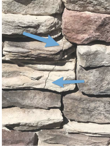
South (Stress Crack)
