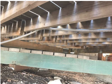
South - Under Deck
