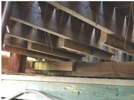
South - Under Deck
