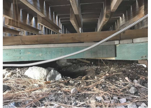
South - Under Deck
