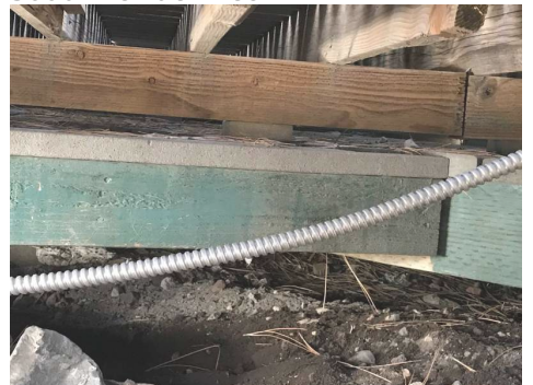
South - Under Deck
