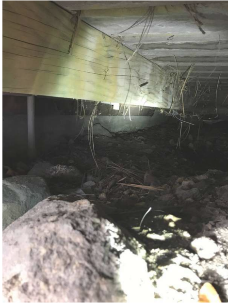
South - Under Deck
