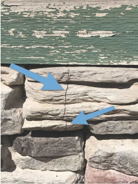
South (Stress Crack)
