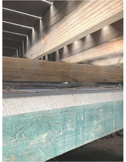
South - Under Deck
