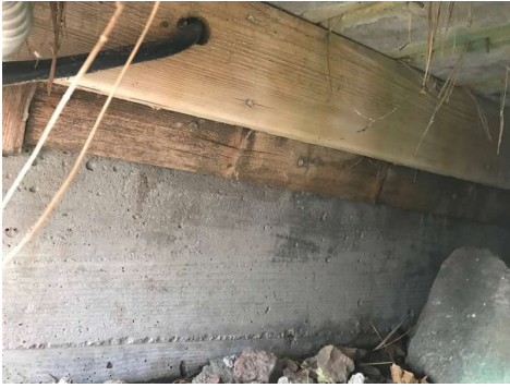
South - Under Deck
