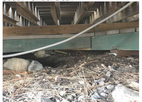
South - Under Deck
