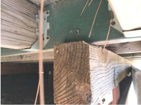
South - Under Deck
