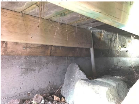
South - Under Deck
