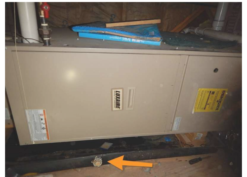
drain for the catch pan has not been plumbed into the household drain
