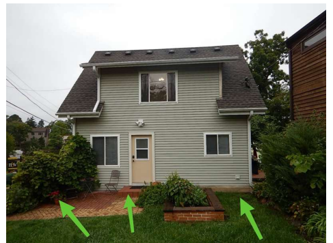
negative grading @ East side of home
