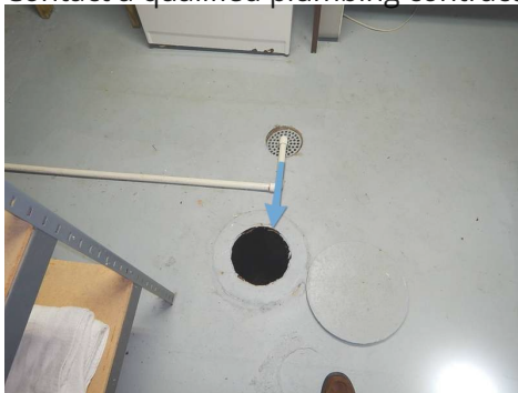
catch basin in use, floor drain is actively discharging to basin
