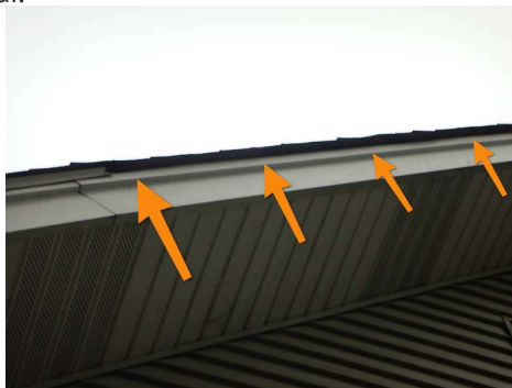
missing section of rake edge flashing
