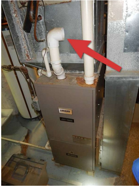
combustion air inlet for high efficiency furnace - recommend obtaining all combustion air from the exterior of the home
