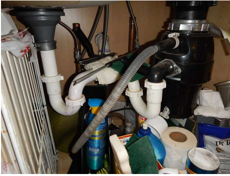
High Loop installation - IL prohibits connections to disposers
