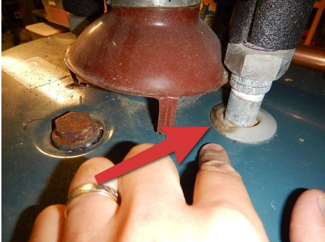
scorching / melting of plastic bushing adjacent to draft collar
