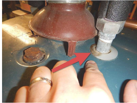
melted and scorched plastic bushing near water heater draft hood, indicative of back drafting condition
