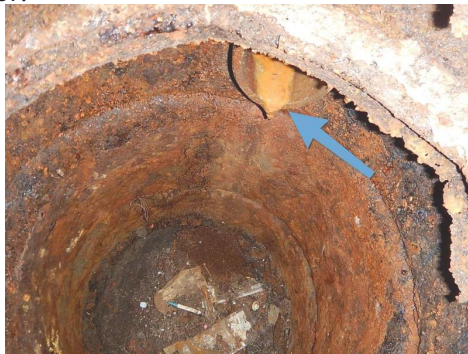
floor drain is actively discharging into a catch basin
