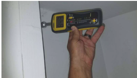
High moisture level at top of closet
