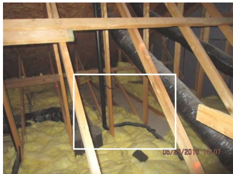
Area in the attic above the master bedroom. Insulation appears to just be tossed aside.
