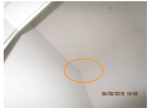
upper corner in closet
