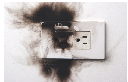
Scorch marks on cover plate
