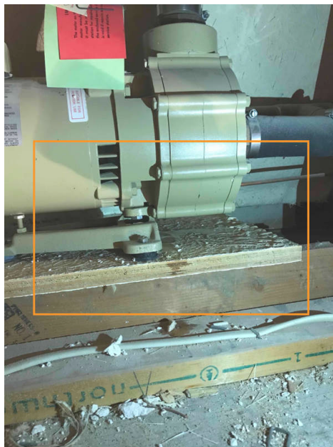
Tub Motor Access in Stairway
