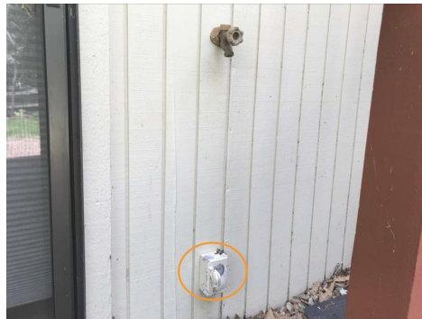
North Side of House on Patio
