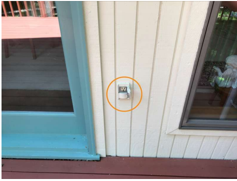
North Side of House on Deck
