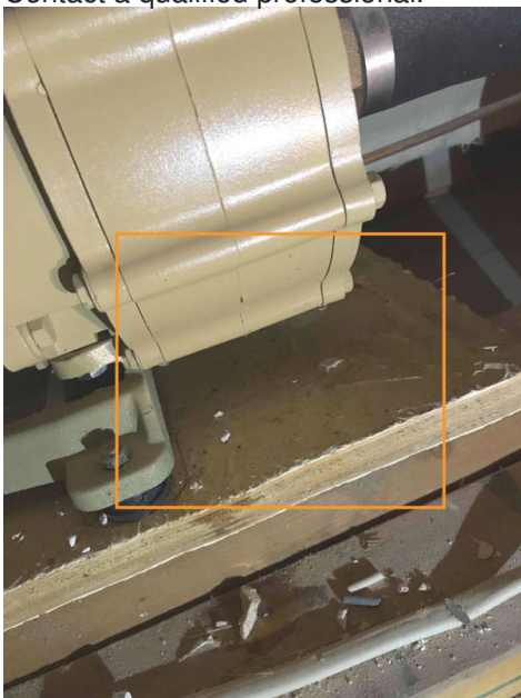
Tub Motor Access in Stairway
