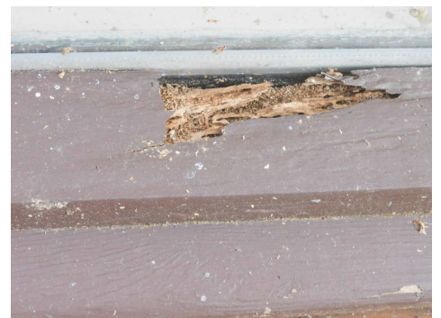
Rear of Home along Deck at Windows
