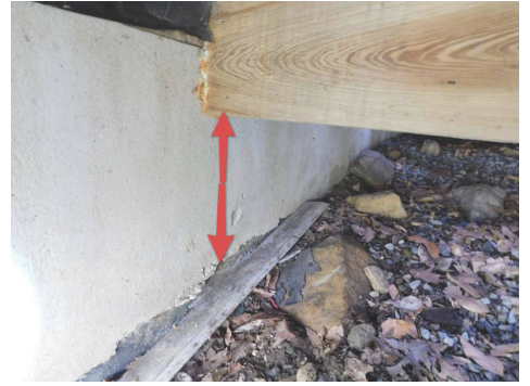
Missing Post Under Support Beam on Deck
