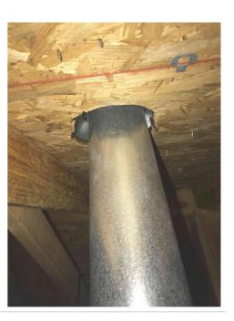
5.3.1 Exhaust Systems BATHROOM VENTS INTO ATTIC
