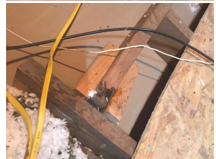
Condensation dripping on framing members.
