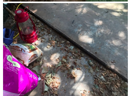
Settling garage slab
