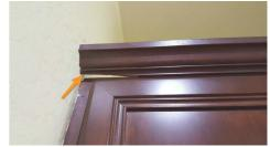
The trim or moulding at the top of the upper cabinets was loose and needs to be re-attached.
