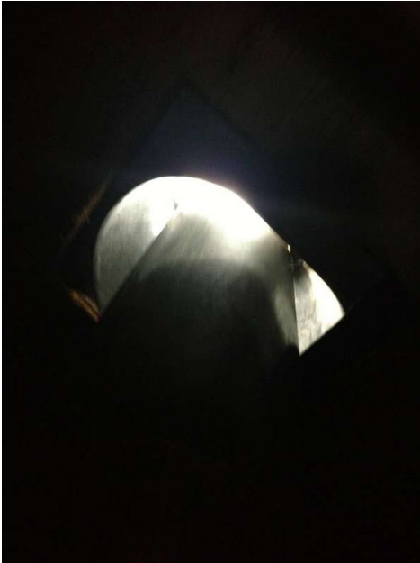
Daylight coming in from around vent pipe.
