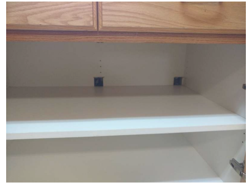
West wall in second floor kitchen.
