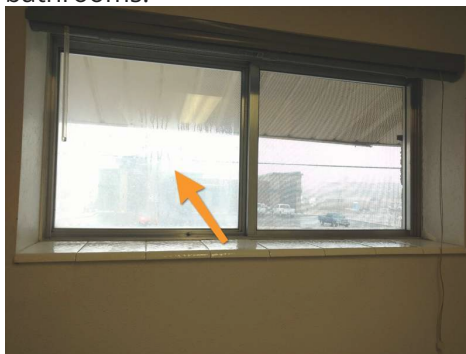
Moisture inside of the window.
