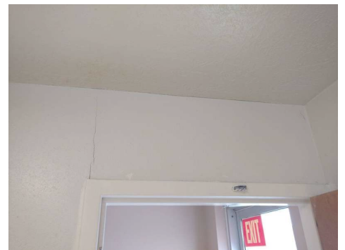
Second floor north bathroom
