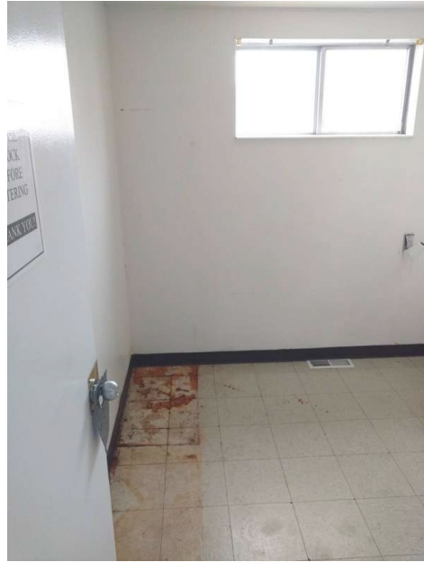
First floor north bathroom
