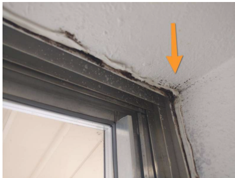
Mold observed around the window in the south bathroom on the second floor. Installing ventilation fans helps mitigate the risk of mold growth in bathrooms.
