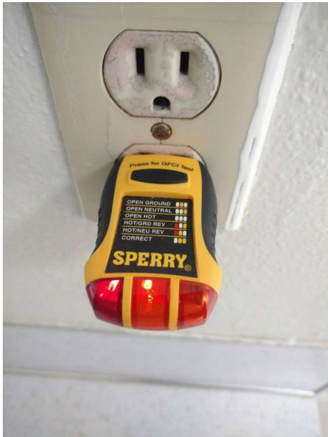
First Floor North Bathroom
