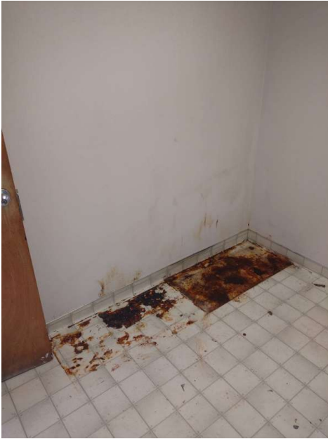
Second floor north bathroom.
