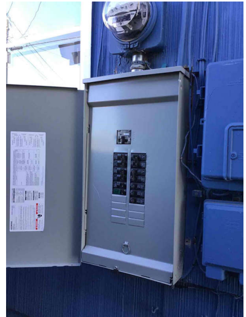
Each circuit should be labeled
