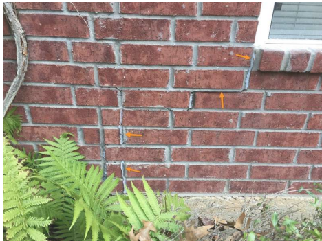
There appears to be rotation of the brick face just below the corner of the window.
