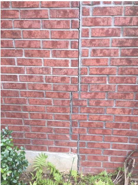
Right rear of house.
