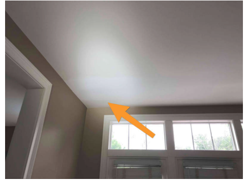
Kitchen ceiling near door to deck has been repainted evidence of a prior water damage incident repair appears proper no further repair required at this time
