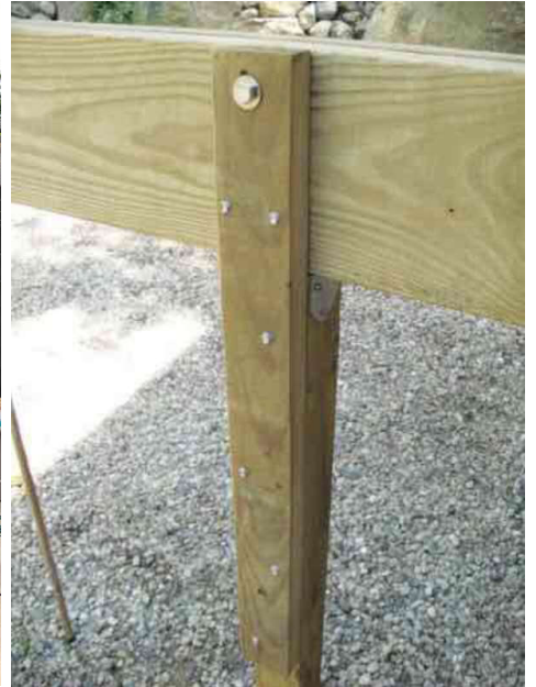
Example photo of a recommended repair for the improper post to beam connections
