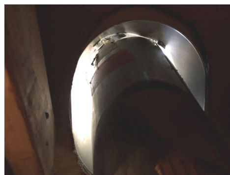
Furnace vent needs exterior flashing
