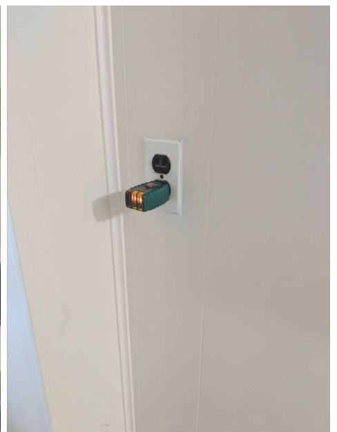
3rd Floor Bathroom
