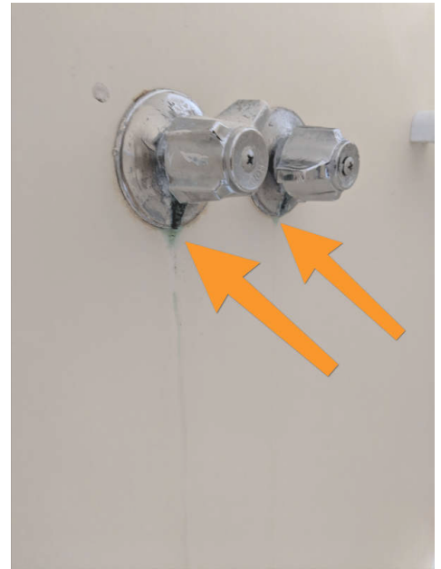
Bathroom 3rd Floor shower
