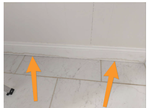
Bathroom 3rd Floor
