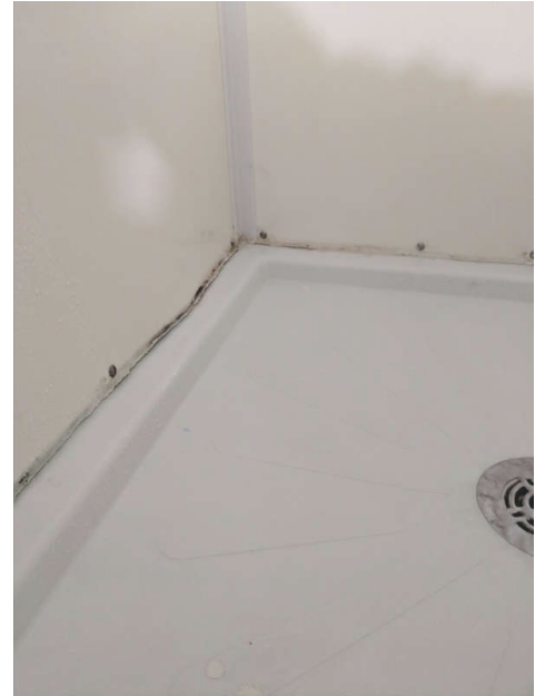
Bathroom 3rd Floor
