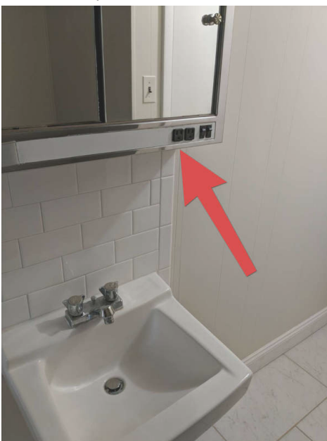
Bathroom 3rd Floor
