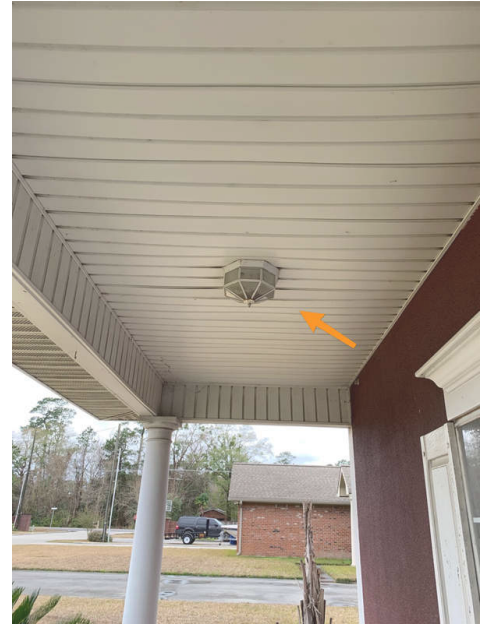
Front of House Garage
