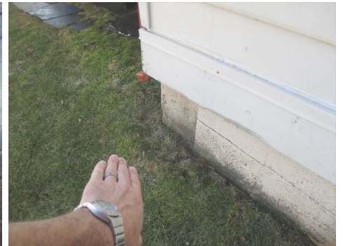
Add downspout extension and improve the grade.
