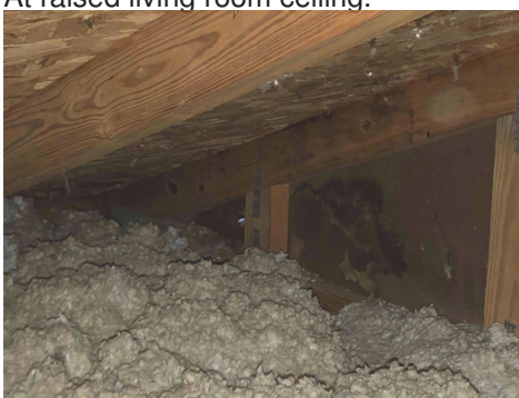
NE corner of attic.
