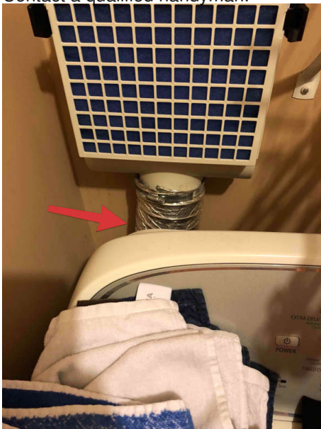
Mylar dryer duct also observed in attic.
