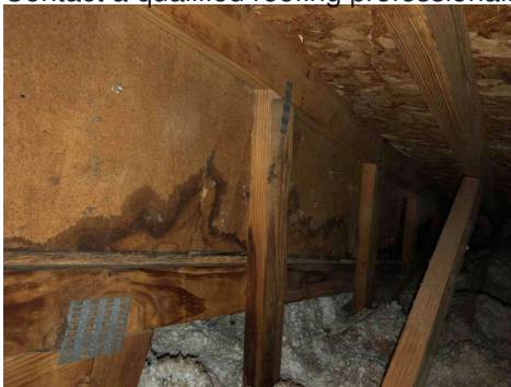
At raised living room ceiling.
