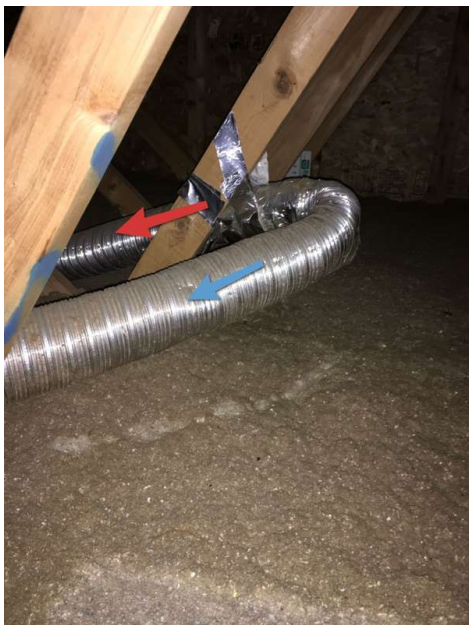
Red To Master Bath : Blue to Second Floor Main
