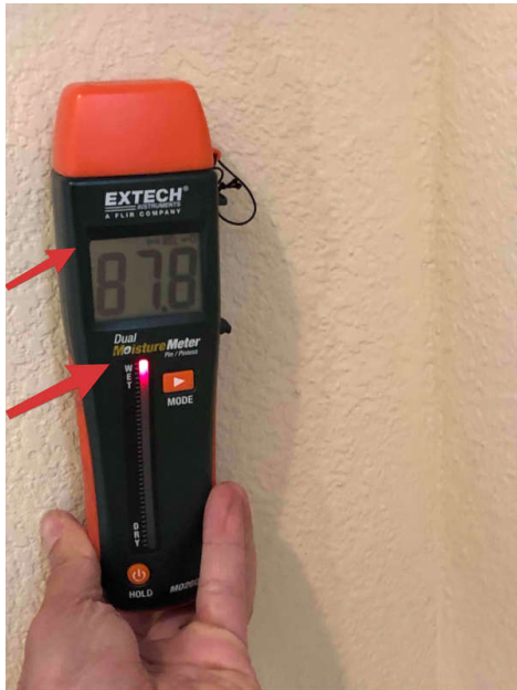
Moisture meter reading
