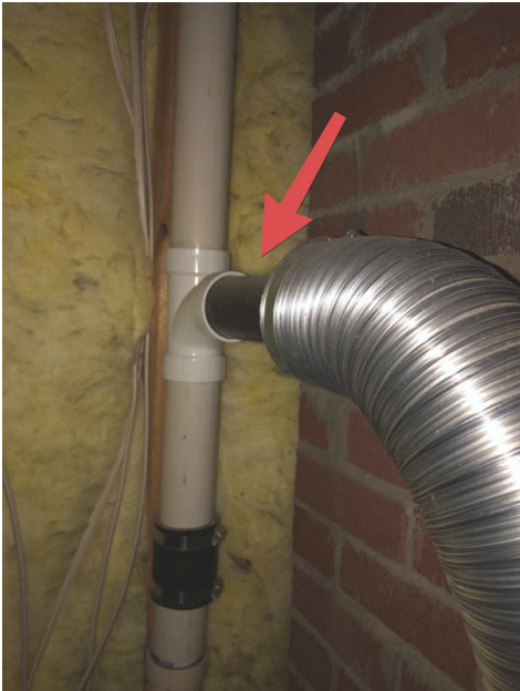
Joining of the two
