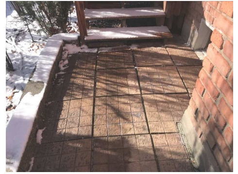
The patio settled on the left side.
