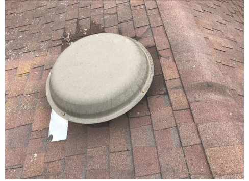
Patching on the attic fan needs to be inspected once a year.
