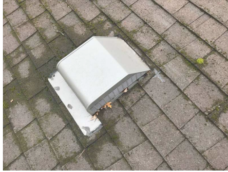
Patching around the vent needs to be checked annually.
