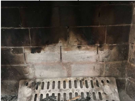
The fireplace in the family room has cracks in the firebox. This is unsafe to use until a level 2 inspection is performed by a chimney sweep.
