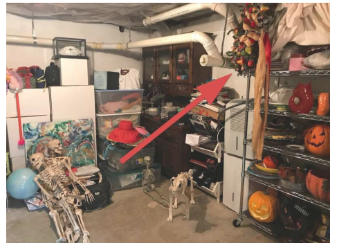
Duct tape is used on the connection where the pipe leaves the building.
