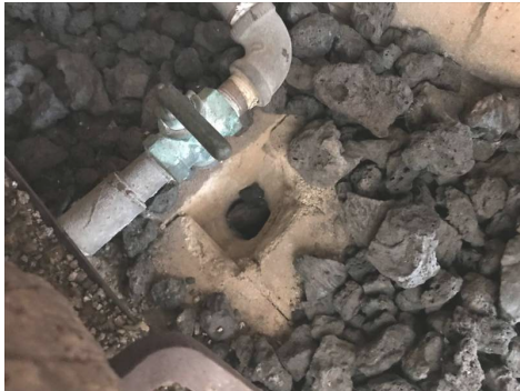
This is the fireplace in the piano room. There is a hole in the floor of the firebox. The isolation valve is inside the firebox.
