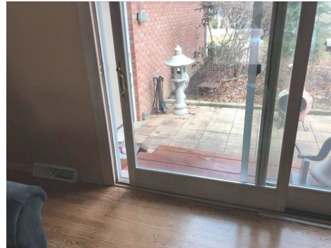
Family room door does not lock
