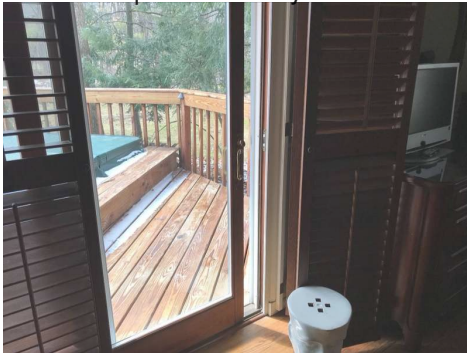
Bedroom door does not lock
