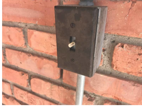
The outdoor dimmer switch is missing a knob
