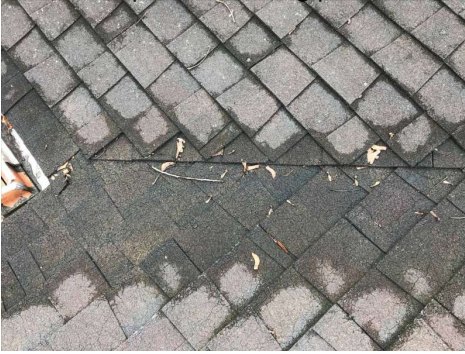
The valley flashing is cracked and worn.
