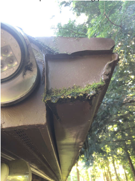
Moss Growing In Leak
