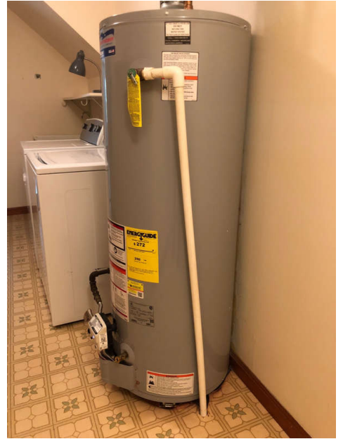
Incorrect TPR Valve
