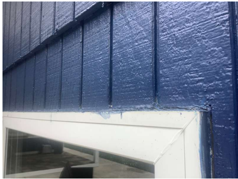
Window flashing detail
