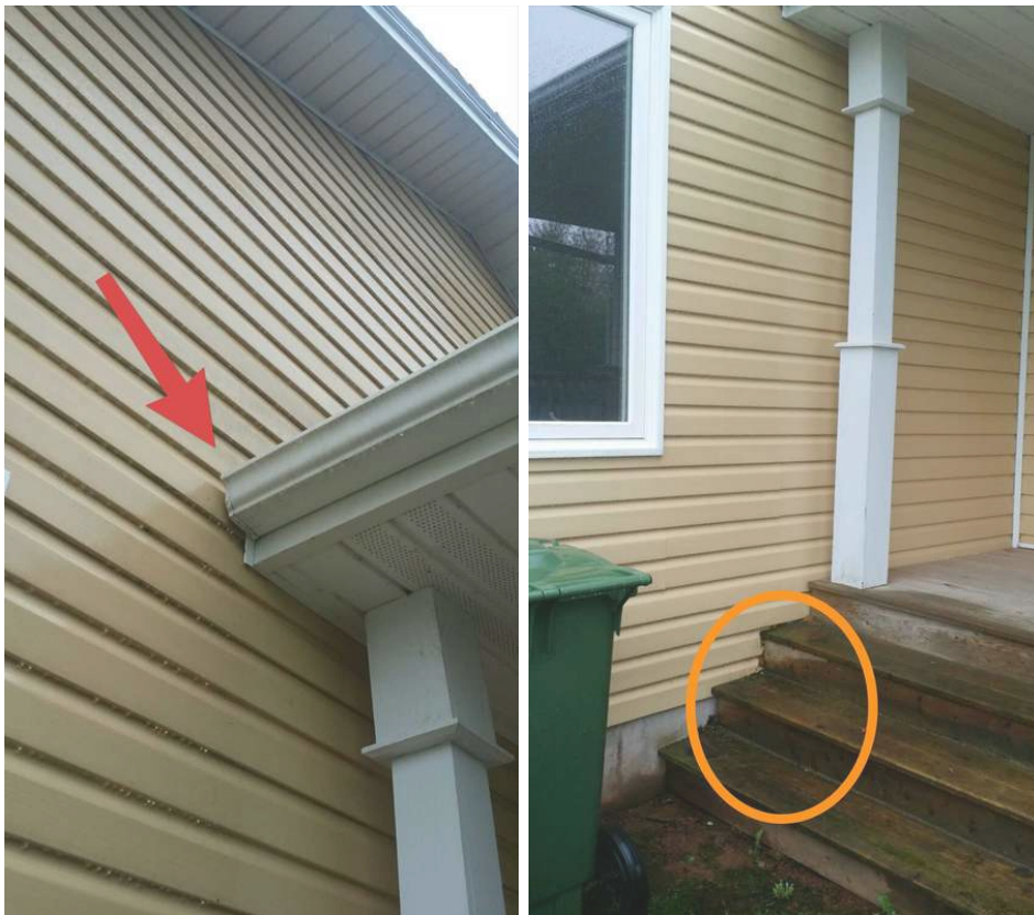
Water over flowing gutter landing on porch steps due to missing Kickout Flashing
