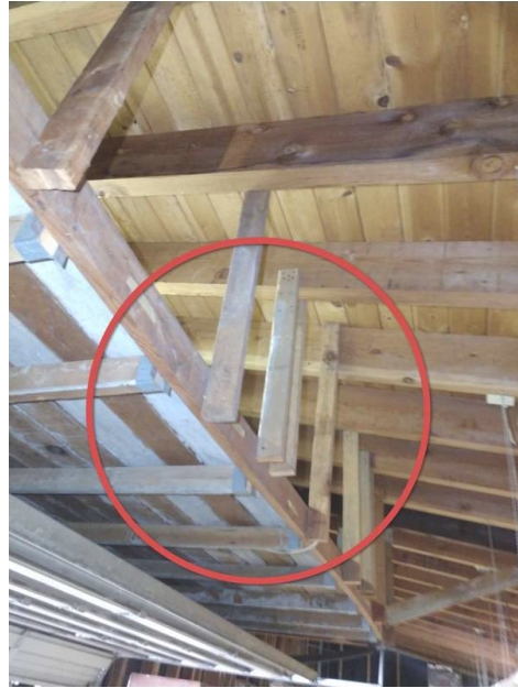
Substandard building practices above garage door.
