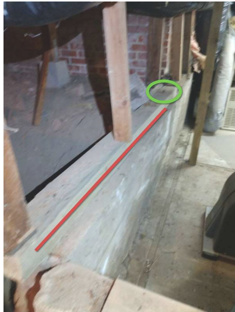
One bolt with no nut or fastener - green circle. No hold down bolts, posts not securely attached - red line
