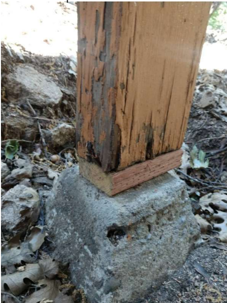
No mechanical fastener securing base to post.
