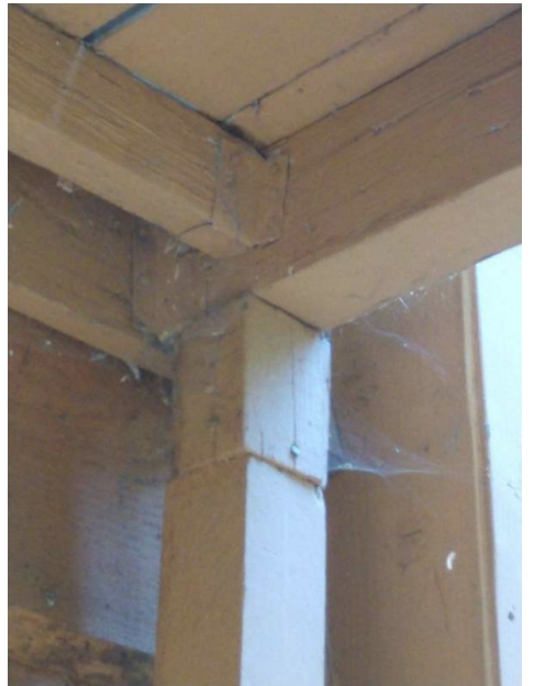
An extension was added to this post supporting the load of a deck.
