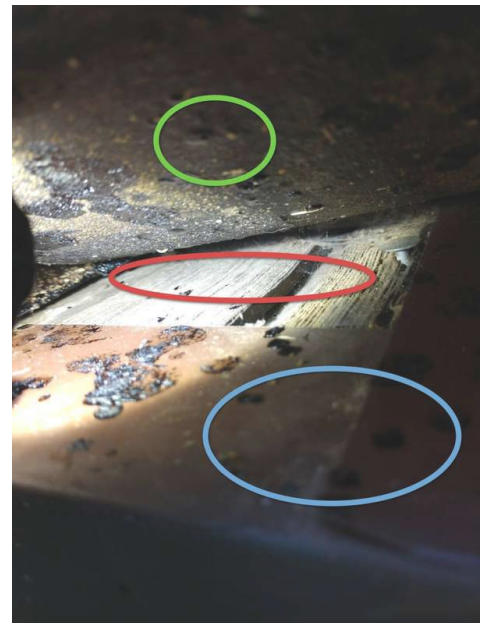
Green circle - bottom of fiberglass shingle Red circle - previous roofing material, wood shingle or shake Blue circle - metal drip edge
