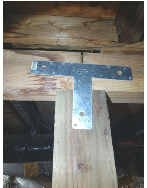
Undersized fasteners for this application.
