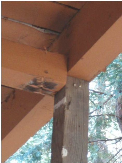
Post is not supporting the load of this framing member.
