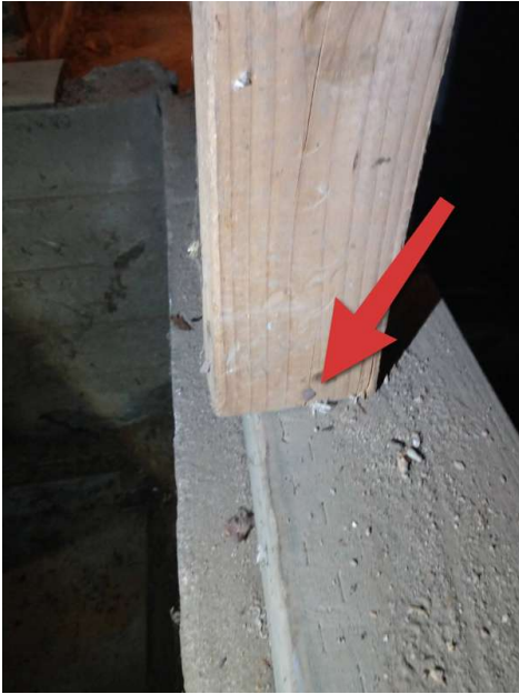
Improper support member, inadequate fastening, poor placement.
