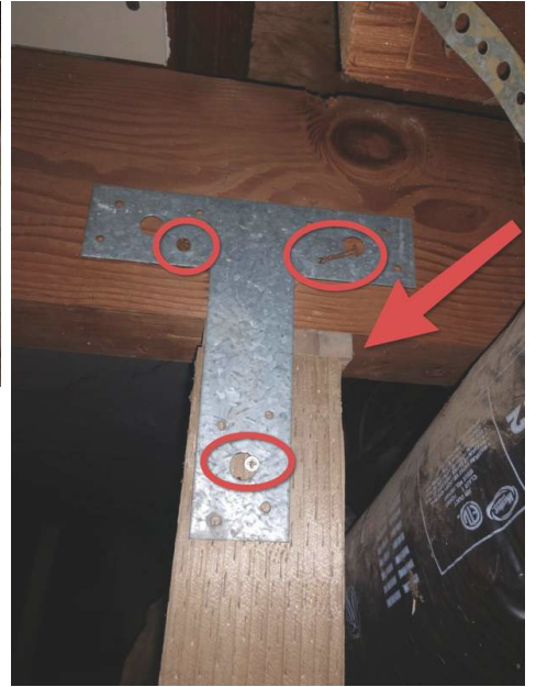
Inadequate number of and improper type of fasteners. Extension / shim inserted.
