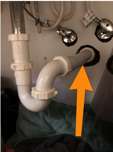
Hall Bathroom sink
