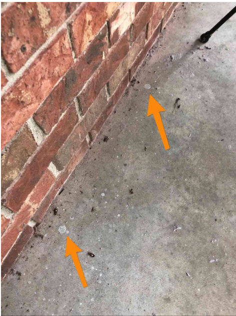
Drill holes- South patio
