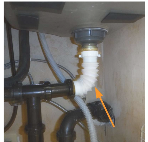
Flex line style drain.
