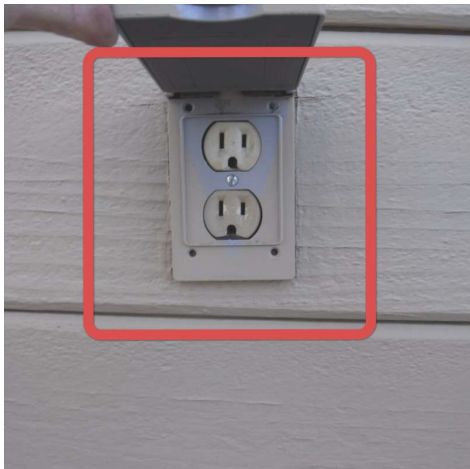
No GFCI at front exterior of house.
