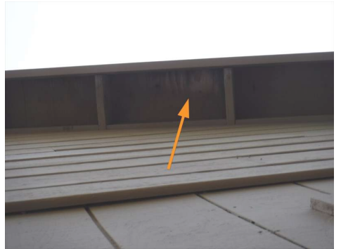
Eave on left side of house
