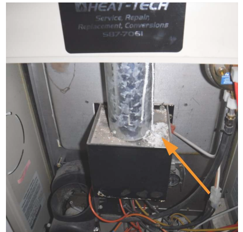
Water entering from gap in roof vent.
