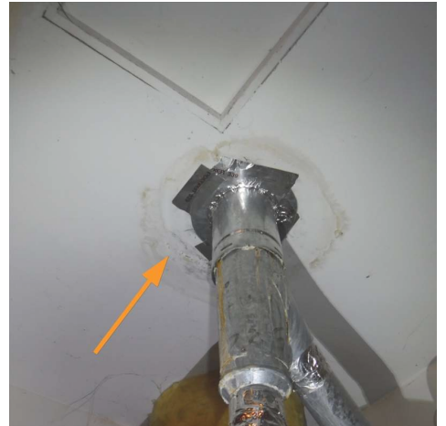
Same vent in garage with ring of water damage.
