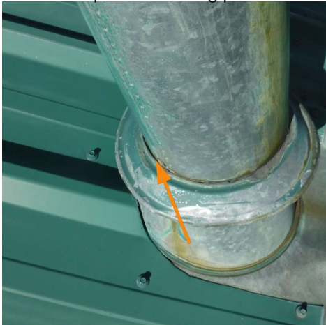
Gap in waterproofing
