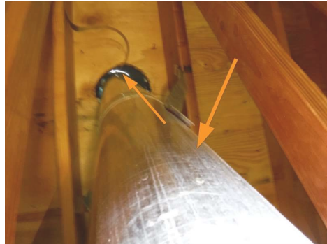
Pipe from inside attic. Water stains from gap in boot.
