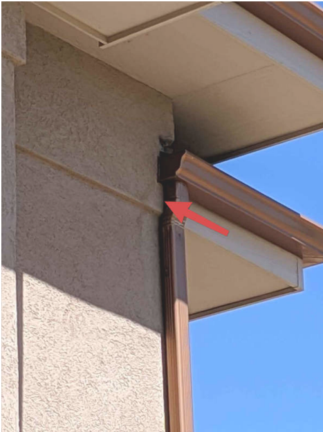
No clear drainage plane
