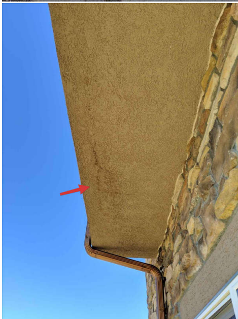
Moisture staining under west window
