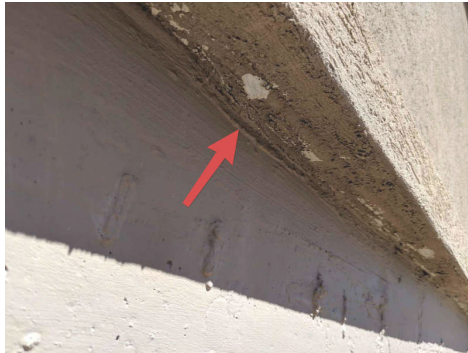
No clear drainage plane
