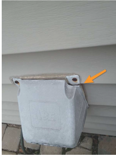
Cracked at top
