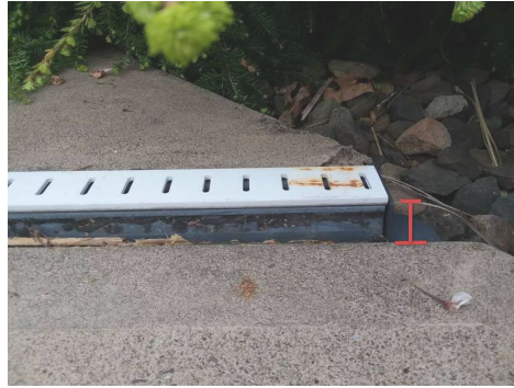
Approx. 1-1/4" difference in height between slabs.
