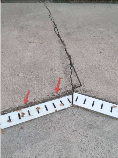
Approx. 3/4" height difference between slabs
