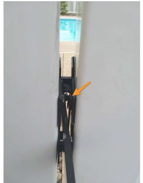
Re-set the post to widen the gap between the post and gate.
