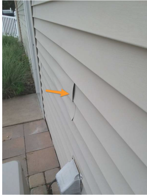
Gap could allow insect intrusion behind siding.
