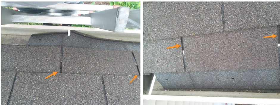
Underlayment exposed at water ways
