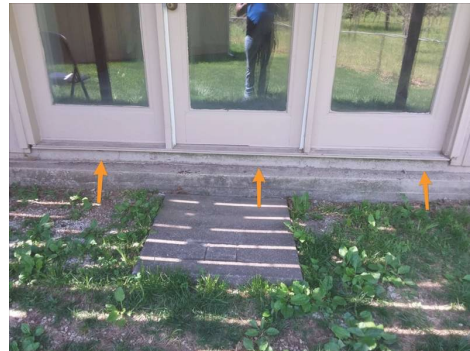
Lower level back door
