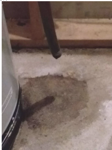
DISCHARGE PIPE ON TPR VALVE
