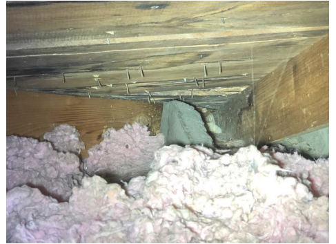
Left Side of Attic Space (above laundry room area).
