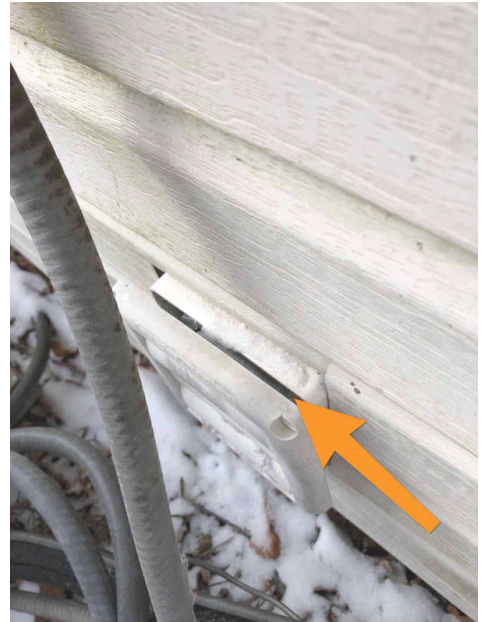
Dryer vent- East
