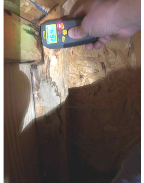
East Garage Attic-near access
