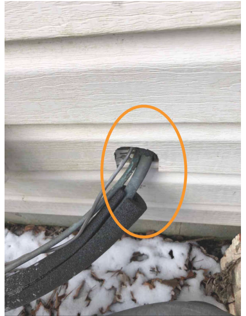
Missing insulation
