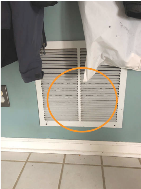
One 16x16 filter 1st Floor
