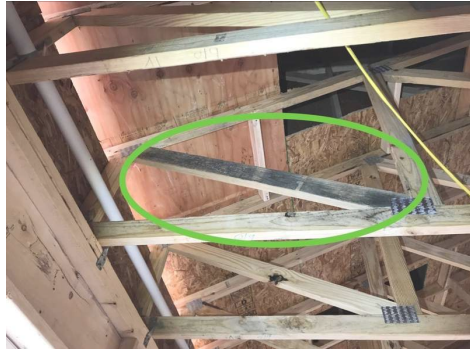
Suspected Mold Above 3rd Floor Bedroom (Front)
