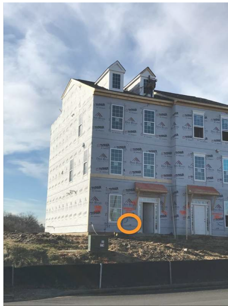
Front Hose Bib Loose
