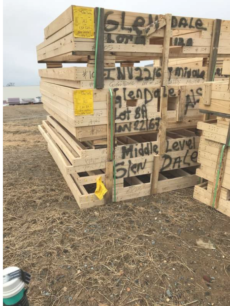
Trusses Stored With Ground Contact / Uncovered
