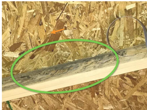
Suspected Mold On First Floor Truss
