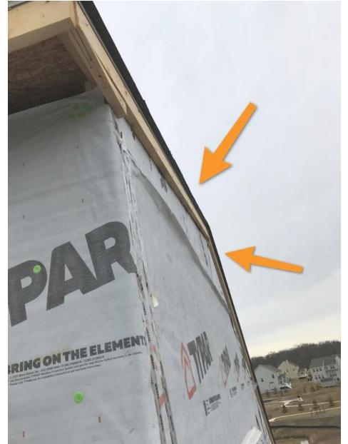
Missing House Wrap Tape
