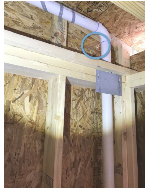
Damaged OSB Sheathing On 4th Floor Exterior Wall
