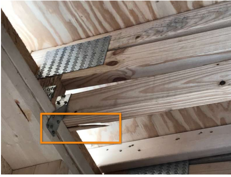
Damaged Chord Truss
