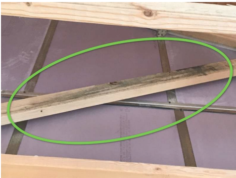
Suspected Mold Above 3rd Floor Bedroom (Front)
