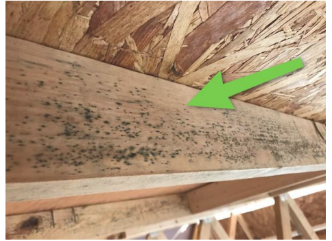
Suspected Mold On Roof Truss
