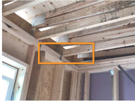
Damaged Chord Truss In Master Bedroom
