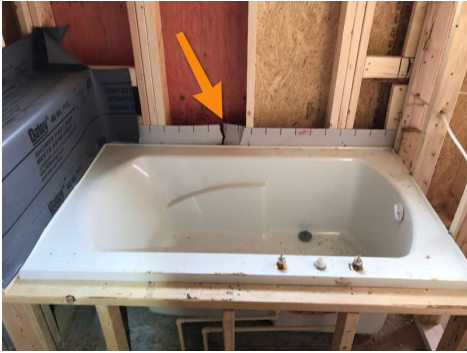
Damaged "Draft-Stop" Rigid Board
