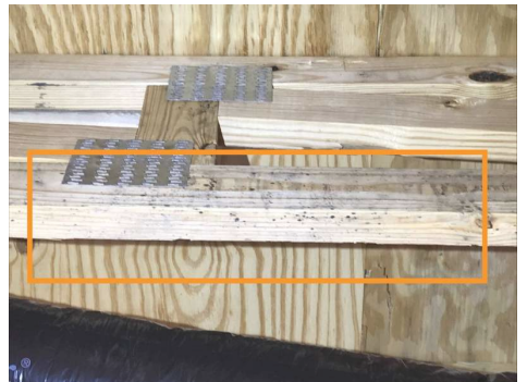
Suspected Mold Growth On Truss Above Master Bathroom
